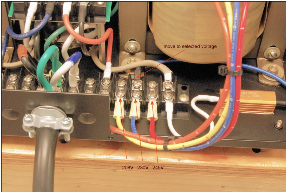
**Figure 14 - Line Voltage Wiring, right side**
